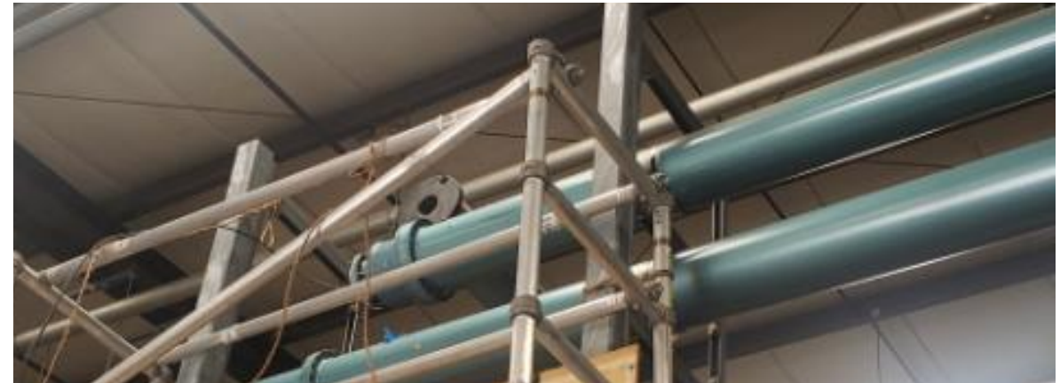
Typical 9" diameter coaxial transmission lines
